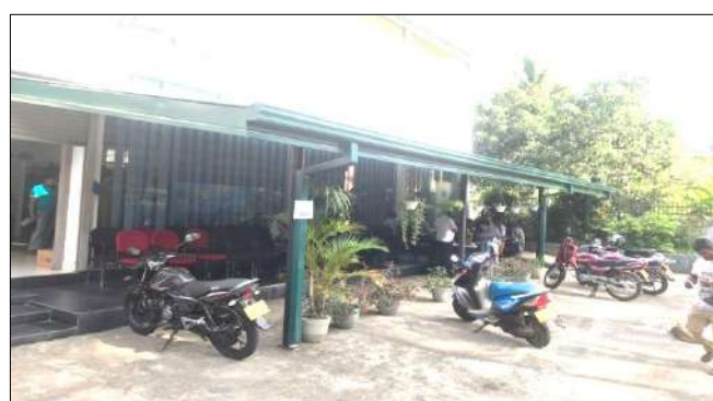
Service Centre at the Kundasale Land Registry
