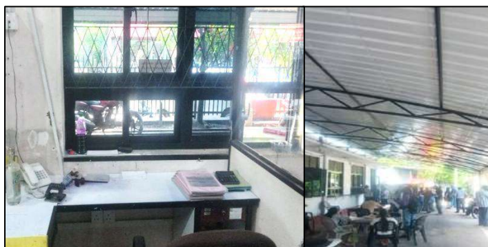
Window Repair Works at the Horana Land Registry
