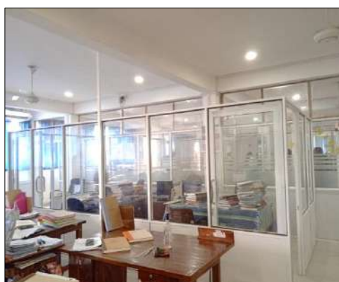
Internal Space Partitioning Works at the Homagama Land Registry Office
