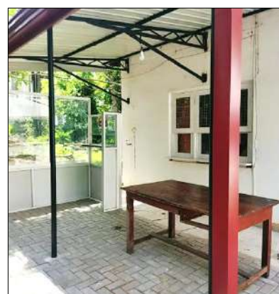
Service Centre at the Panadura Land Registry
