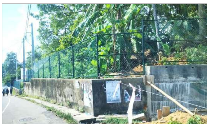
Installation of a Security Fence at the Tangalle Land Registry Office
