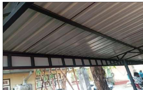
Construction of a Rain Shelter at the Matugama Land Registry Office
